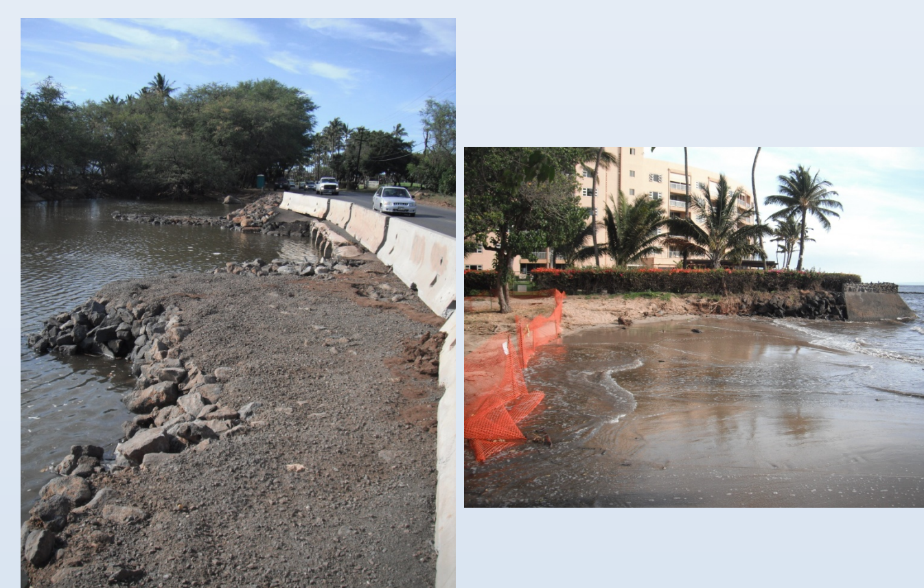
In Kihei, Maui, a rainier than normal La Niña winter season in January of 2011 coupled with intense storms caused beach erosion while flooding damaged road infrastructure. Photos by Victoria Keener.
