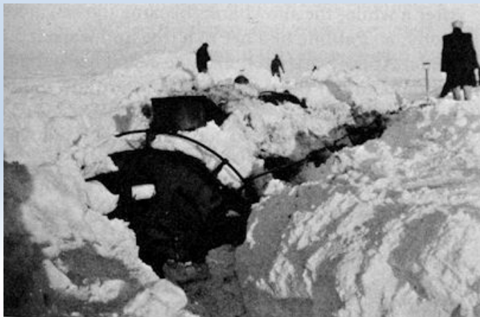
A buried locomotive near Alliance, Nebraska
