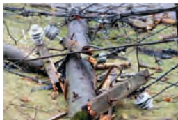
March 12-15, 2010 Downed utility pole and tree branches in Westchester County, NY Source: James Estrin / New York Times
